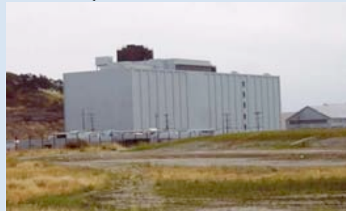
The NRDL beside the scorched Parcel E landfill.
